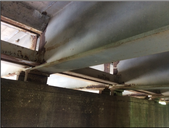
Girders 2-4 @ Bent 6 (corrosion)
