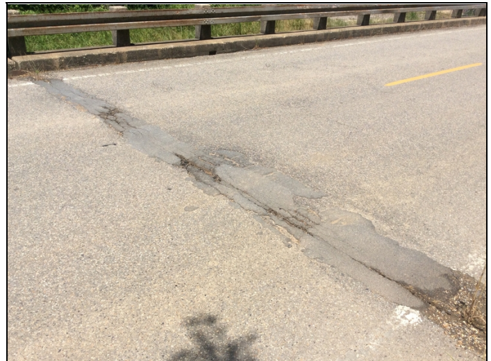
Wearing surface - Bent 6 (cracking)
