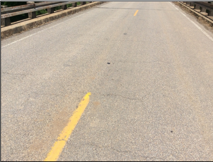
Wearing surface - Span 4 (cracking)
