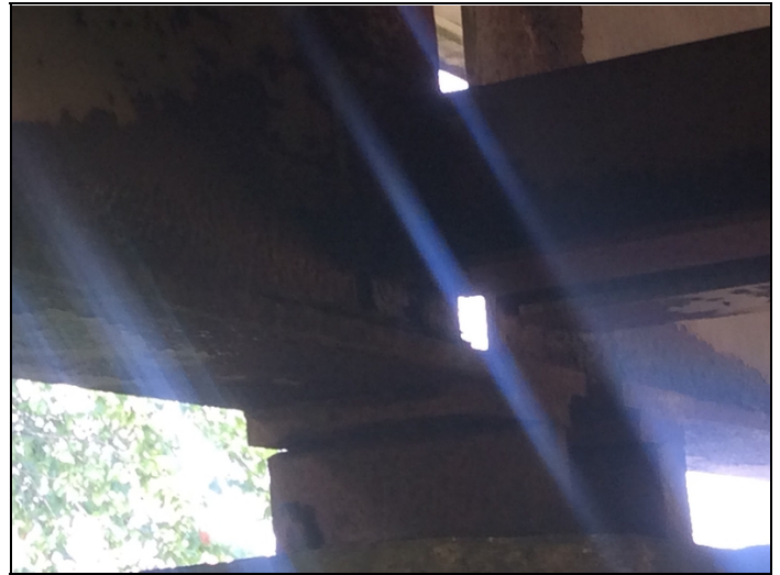
Span 6 at bent 6 girder 5 has flaking rust at bearing area 5'. Common several girder ends this bridge.
