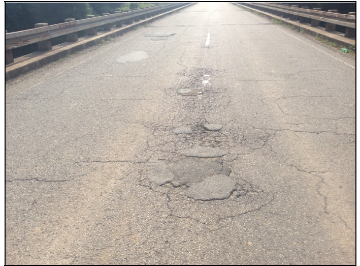
Span 2 wearing surface has patched areas. Common in span 3.
