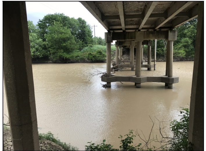
Bents 3-5 has one debris on pile.
