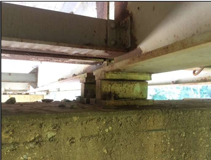
Bearings 2 @ Bent 6 (corrosion)
