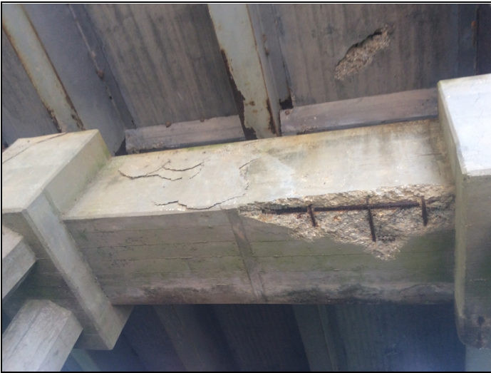
Bent 6 cap has spalls ,delambs and exposed rebar with minor section lose.
