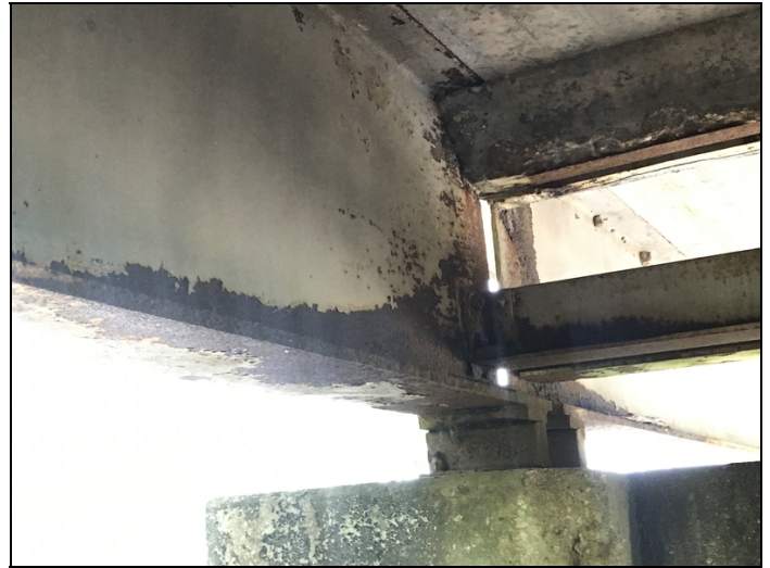
Bent 6 back and ahead, girders hav rust and rus its flaking areas.
