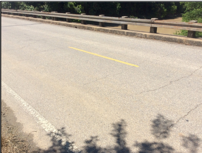
Wearing surface - Span 5 (cracking)
