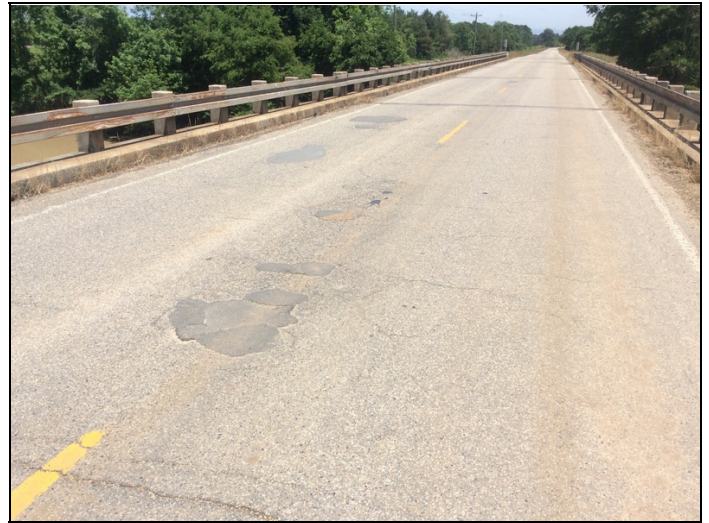
Wearing surface - Span 2 (patches)
