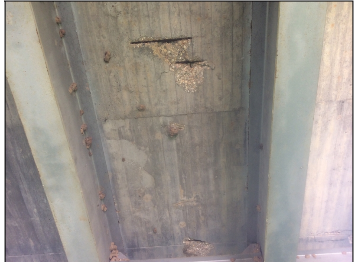
Soffit spalls with exposed rebar common most spans.
