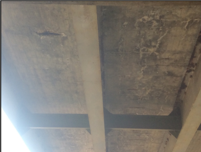
Span 2 soffit spalls with rebar exposed and cracking with efflorescence.
