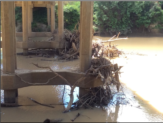
Channel - Bents 3-5 (debris built-up)
