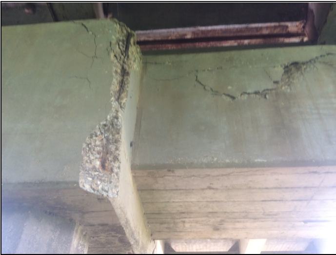
Bent 2 cap under girder 3 has spalls, delambs and exposed rebar .
