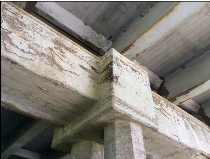
Cap - Bent 6 back (delamination)
