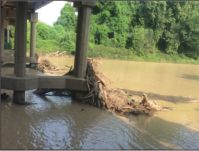
Drift and debris at bent 4&5 on piles 1&4 at each bent.
