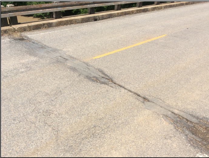
Wearing surface - Bent 4 (cracking)
