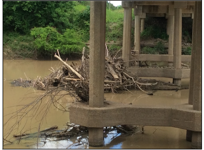
Channel - Bents 3-5 (debris built-up)
