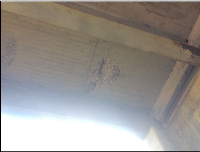
Span 5 under side of deck has spalls with exposed rebar between girders 1&2 near bent 6 .
