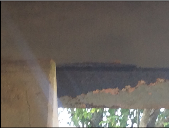
Span 5 at bent 6 at girder 5 has heavy flaking rust .
