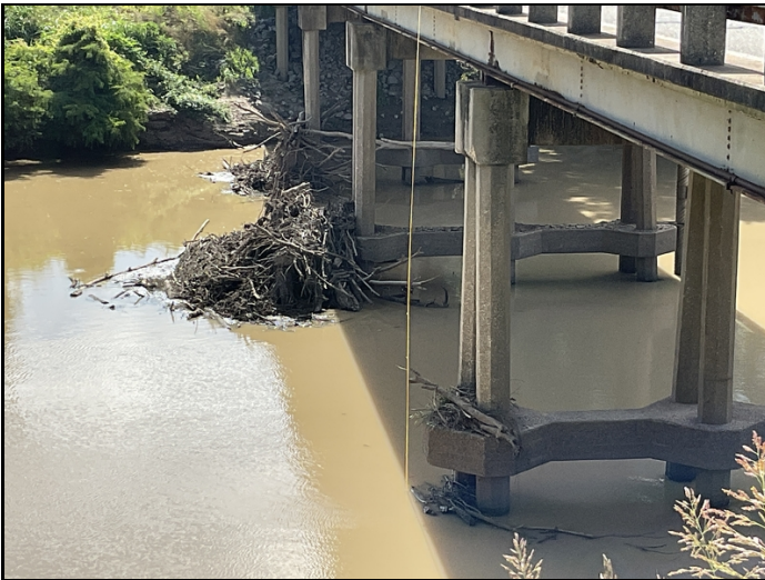
Channel - Bents 3-5: Debris build-up
