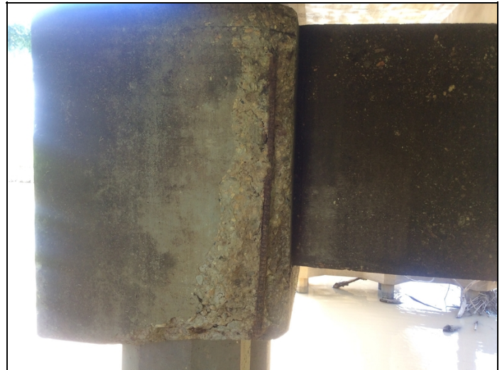
Cap - Bent 6 right ahead (rebar exposed)
