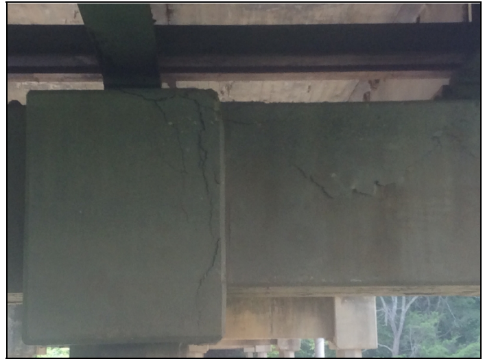
Bent 2 cap back has spalls ,spalls with exposed rebar and delaminations. Common ahead face and bents 3,4, 5 & 6.
