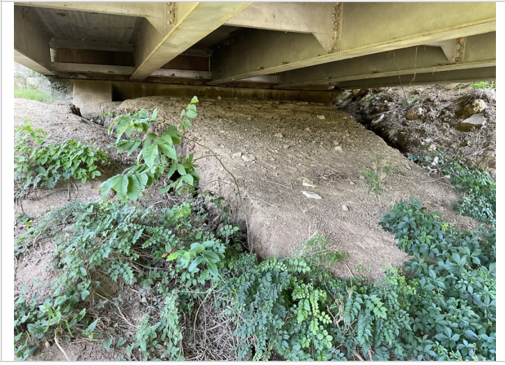
End-slope - Bent 1: Erosion
