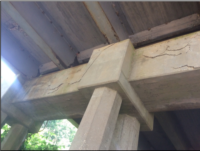
Bent 6 cap ahead face has heavy delambs .
